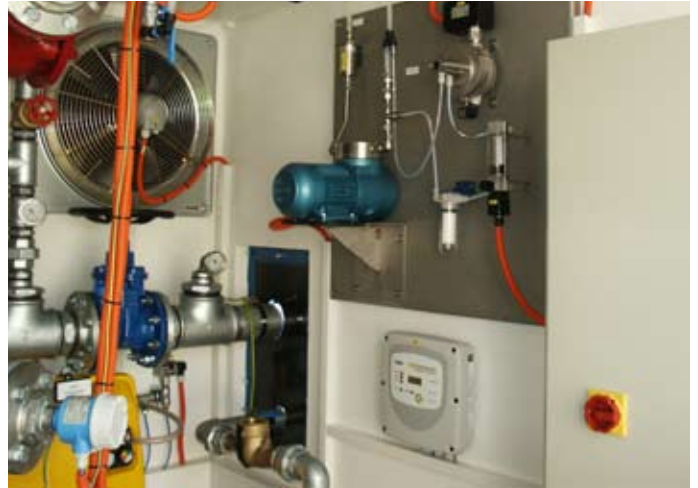
HVE-container with blowers, liquid separator and control panel
