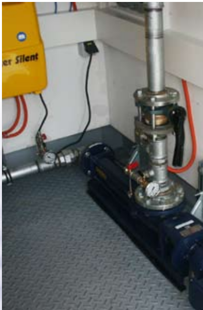
Discharge pump of the liquid separator
