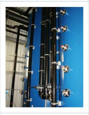
Sand filter equipped with automatic backwashing; plant is equipped with process visualisation and remote control
