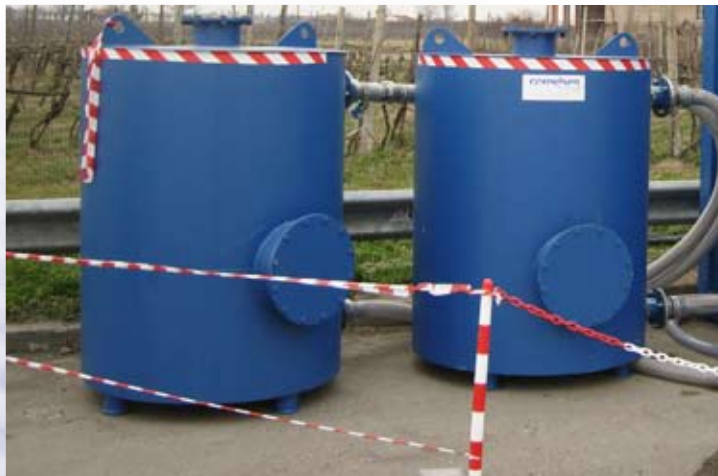
Plant installed in a 20 ft container at the edge of a service area; 2 vapour phase carbon vessels made of steel installed outside the container
