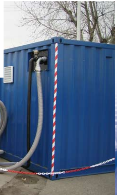
4 header lines connecting the MPE wells to the inlet coupling of the container
