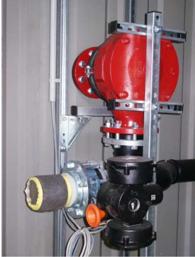
LEL detection system (inline) and liquid separator (detonation proof)
